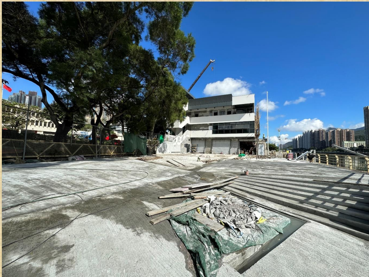
Boat House - Open Yard area as of 29 th November
